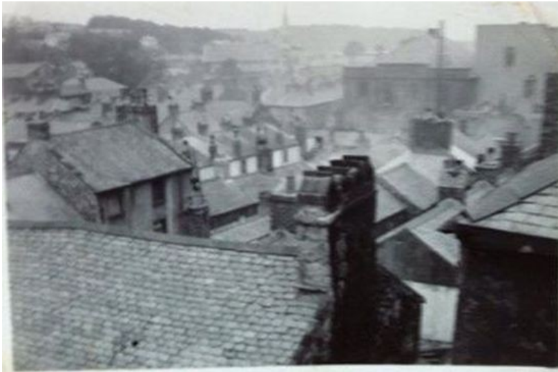
Taken from the rear of a High Street property with the roof and chimney of the Three Crowns pub, foreground left, County Theatre in the distance and London House foreground right.
